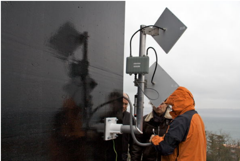
Figure 8: Assembling of node01 on the platform roof of the University of Neuchâtel.
