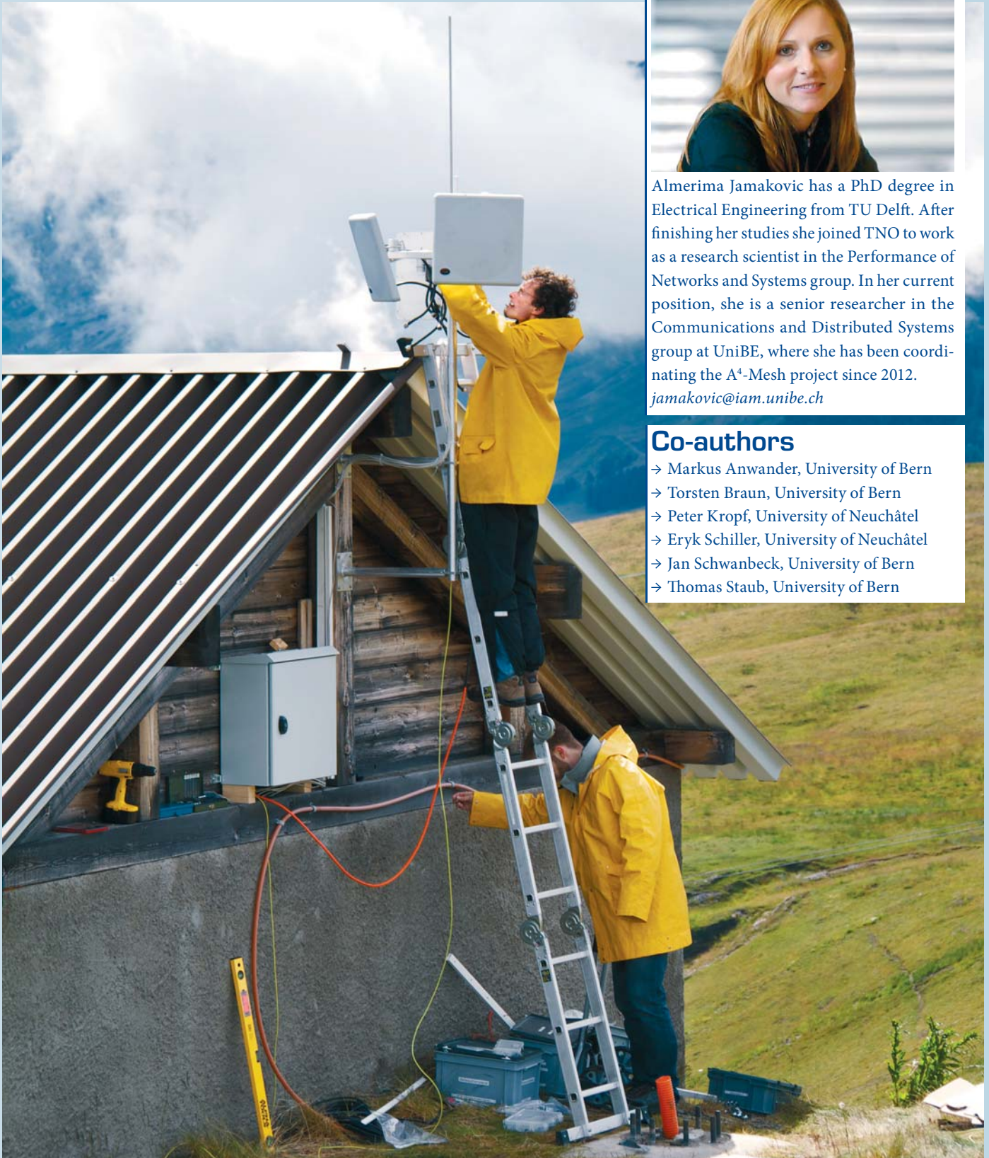
Installation of an in-field mesh node for environmental research in the Valais region.
